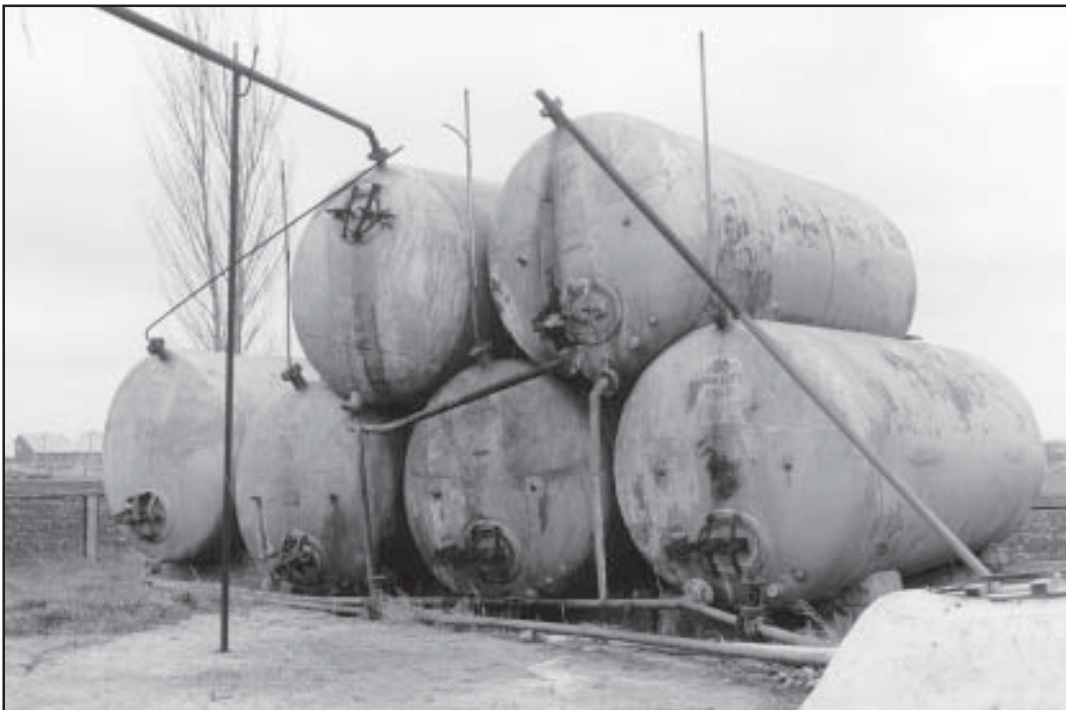
Tatarbunary: tanks with drinking water at the emergency storage
