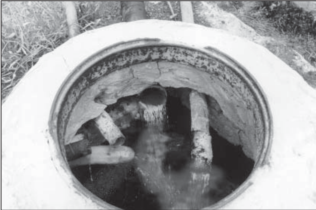
Hole of the main drinking water reservoir at the Tatarbunary pumping station in deterioration
