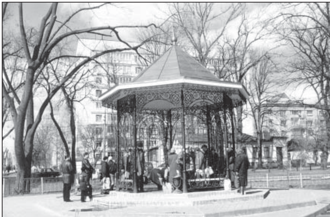
One of 70 pump rooms with artesian water operating in Kyiv
