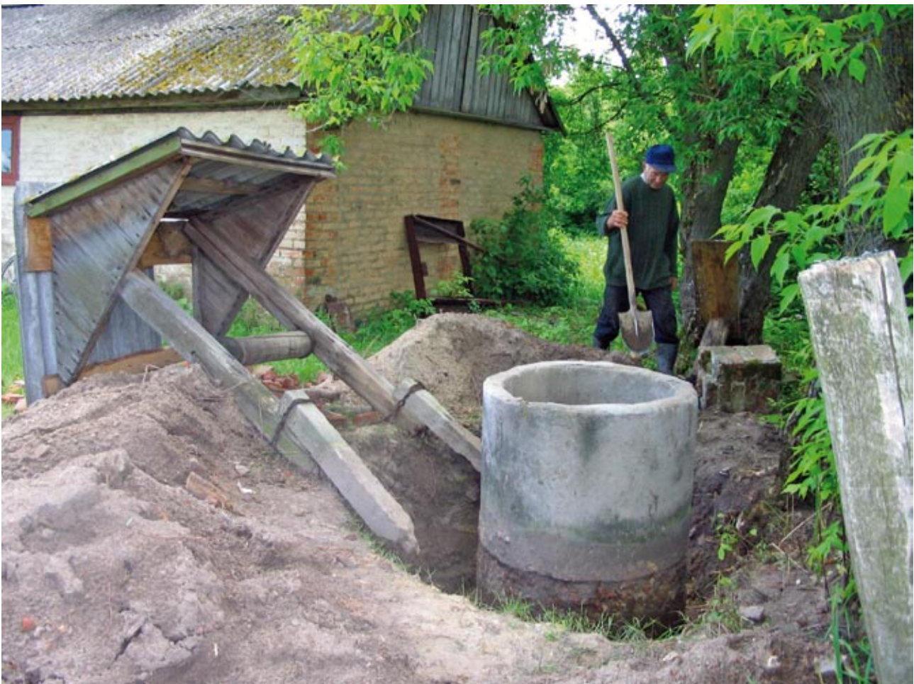
Photo 15. Drinking water well reconstruction in v. Bobryk, Chernigivska oblast
