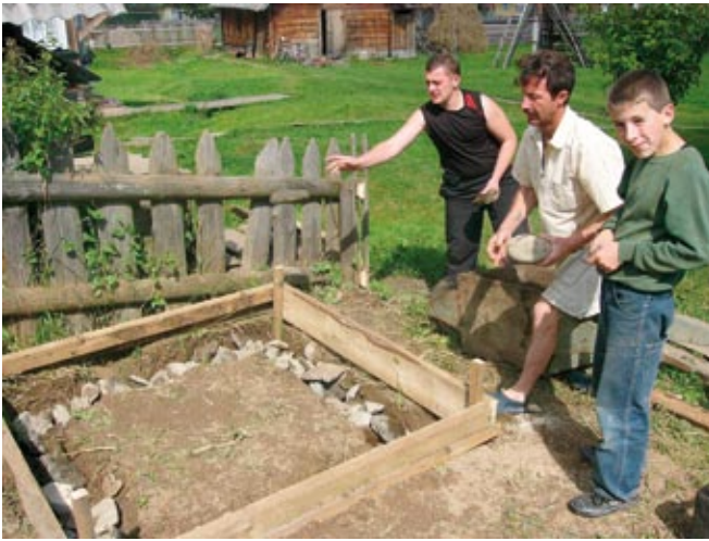
Photo 8.1—8.4. Building the ecosan-toilets in Vorokhta township, Ivano-Frankivska oblast
